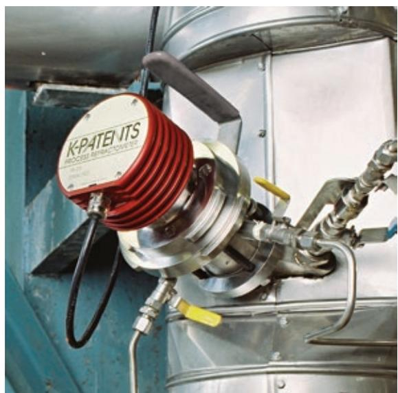
SAFE-DRIVE® PROCESS REFRACTOMETER PR-23-SD
